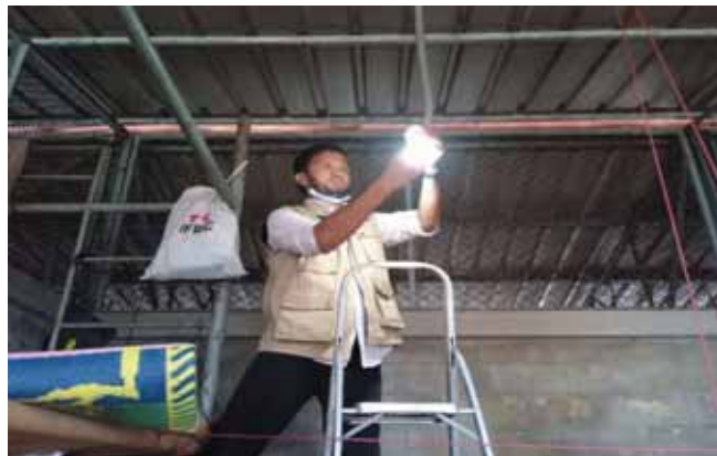
Repairing Solar light at Cluster-86. 22.03.23. Photo: Md. Rashid.
