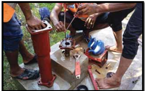
Water point repairing at Cluster 85. 04.11.22, Photo: Abul Hossain.
