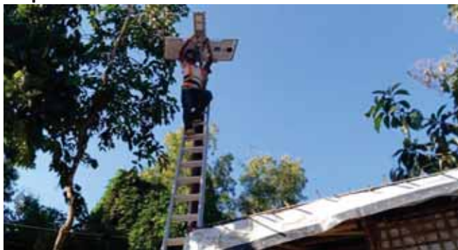
Adolescent Saddam is working on installing street solar lights along the road in the camp under IOM organization. Pic- Md Lokman, FC, Camp- 14
