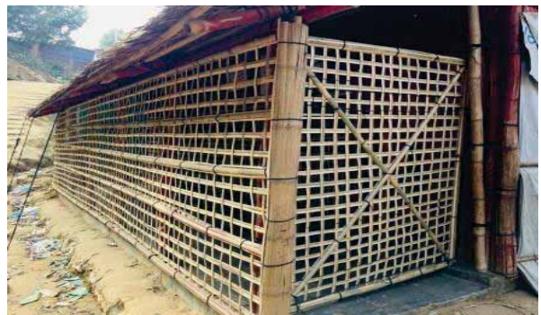
Safe LC, after renovation work, Photo by: Alam Badsha
