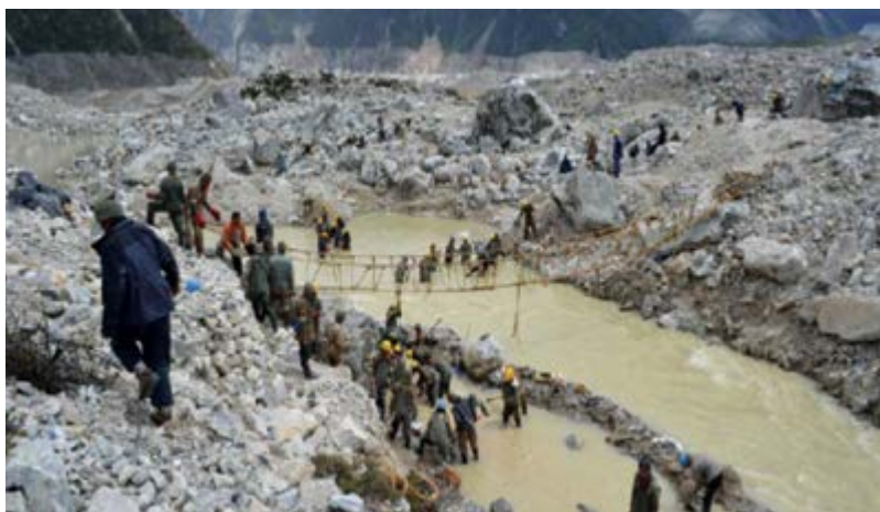
Figure 9: Risk reduction method to avert GLOF includes artificially lowering the water level of the lake through human intervention
