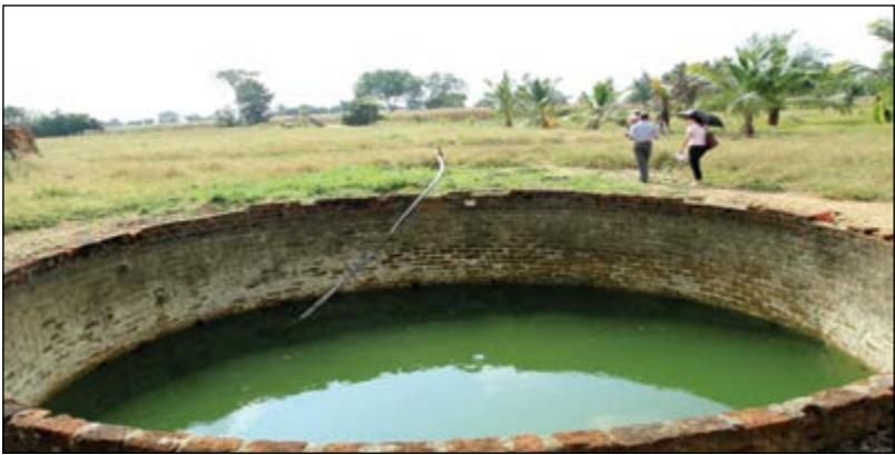
Figure 1. A typical lined agro-well in the authors' study area.
