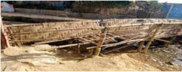
Learning centre come and out pathway bamboo broken Bridge. Pic: Suraya (PO)
